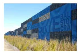
With construction of the M5 Freeway in New South Wales, Qenos provided Alkatuff<sup>®</sup> LL711UV polymer for the sound wall panels to be rotomoulded by Viscount into 6 m lengths, up to 600 mm high and 30 mm deep, with a UV requirement of 18 years. Over nine months, 15,000 individual panels were installed across 18 km.
